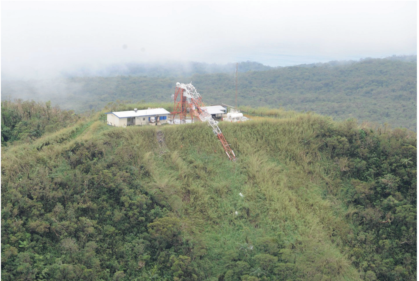
Damaged Telecommunications Tower after Tropical Cyclone Winston (Source: Pratarp Singh)
