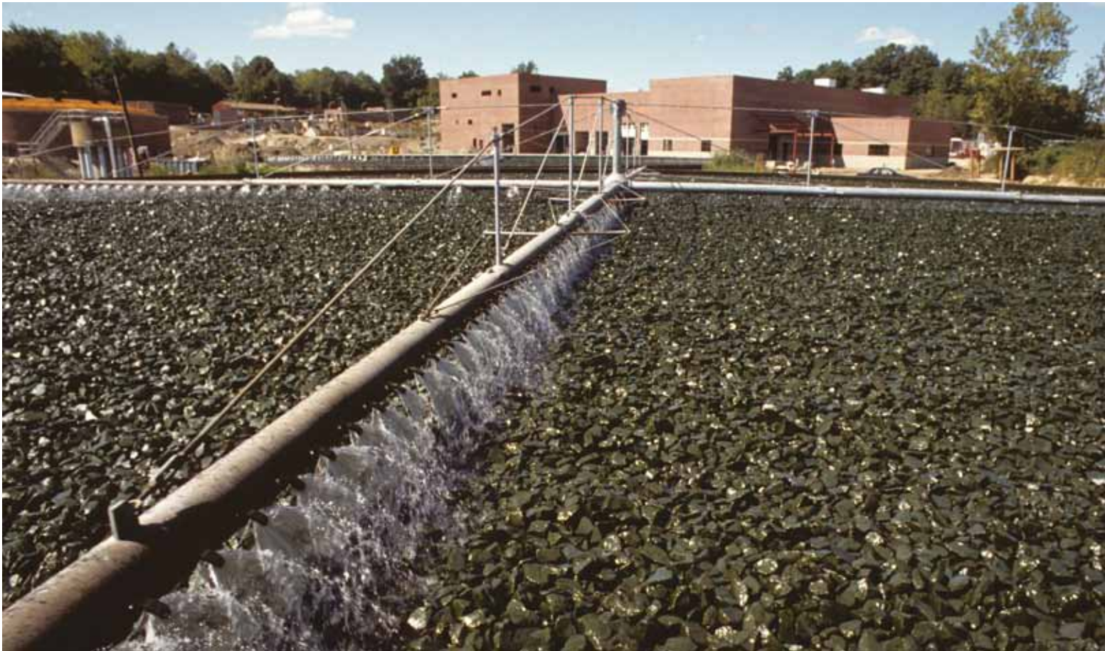
Fig. 6. Treatment Plant Wastewater. Danbury, Connecticut, USA. © UN Photo/Evan Schneider.
