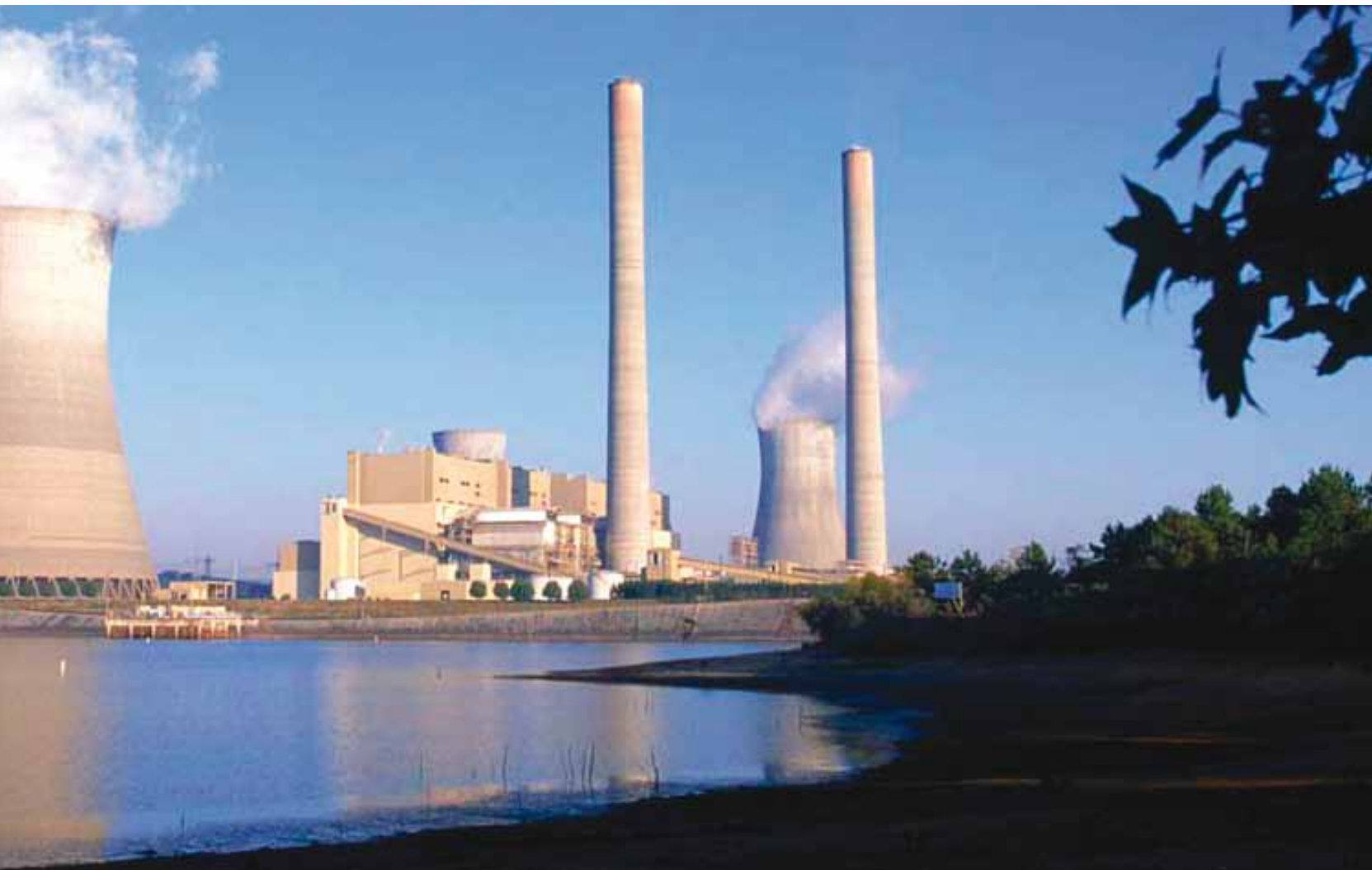
Fig. 5. Plant Scherer, a coal power plant in Georgia, uses a closed loop cooling that removes significantly less water than a one-step system.
