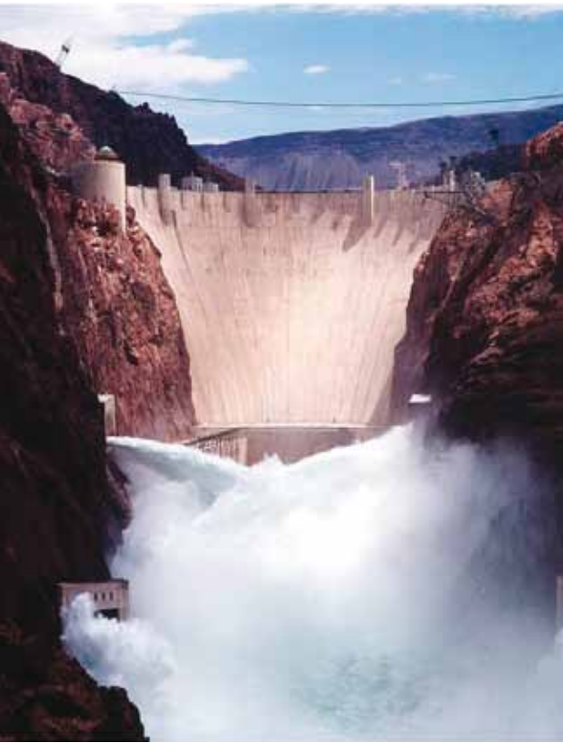
Fig. 6. Hoover Dam releasing stored water for other uses downstream.
