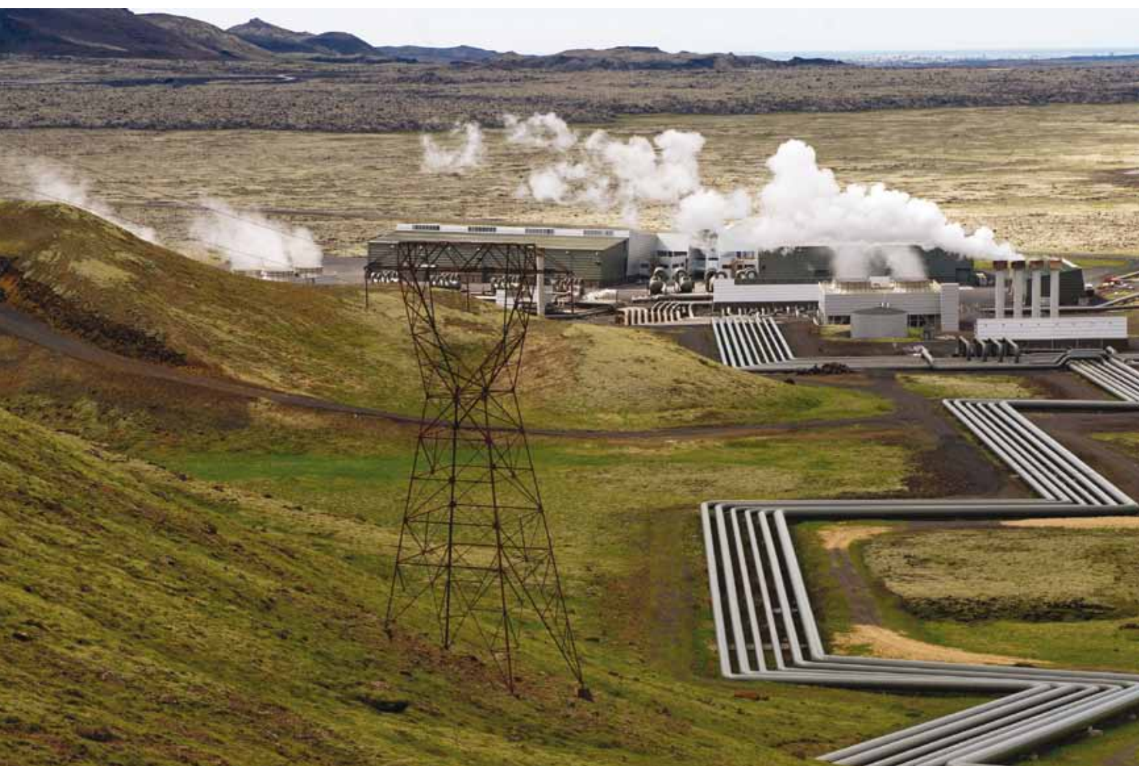
Fig. 3. Hellisheidi geothermal power plant in Iceland. Located in the Hengill area, an active volcanic mountain range in southwestern Iceland. Hengill, Iceland. © UN Photo/Eskinder Debebe.
