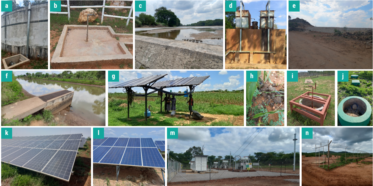
Figure 8: (a) Ongoing expansion of Esigodhini water treatment and supply system; (b) a private sector-funded community water supply scheme; (c) a sand dam at Tuli; (d) a sand dam water treatment and supply system at Ntepe; (e) ongoing construction of the Tuli-Moswa Manyange multi-purpose dam; (f) a dam supplying water at Mzinyathini irrigation scheme; (g, h) a solar-powered, drip-irrigated and organic manure fertilized community food and nutrition garden at Esibomvu; biogas digesters (i) supplying fuel for cooking and treated manure at a livestock farm and (j) energizing at Gwanda Agricultural Show; and solar power farms (k) in construction at Richaw site in Gwanda, (l) energising Mashaba community, (m) energising Blanket (Caledonia) Mine, (n) and in construction at Intratek site in Gwanda.
