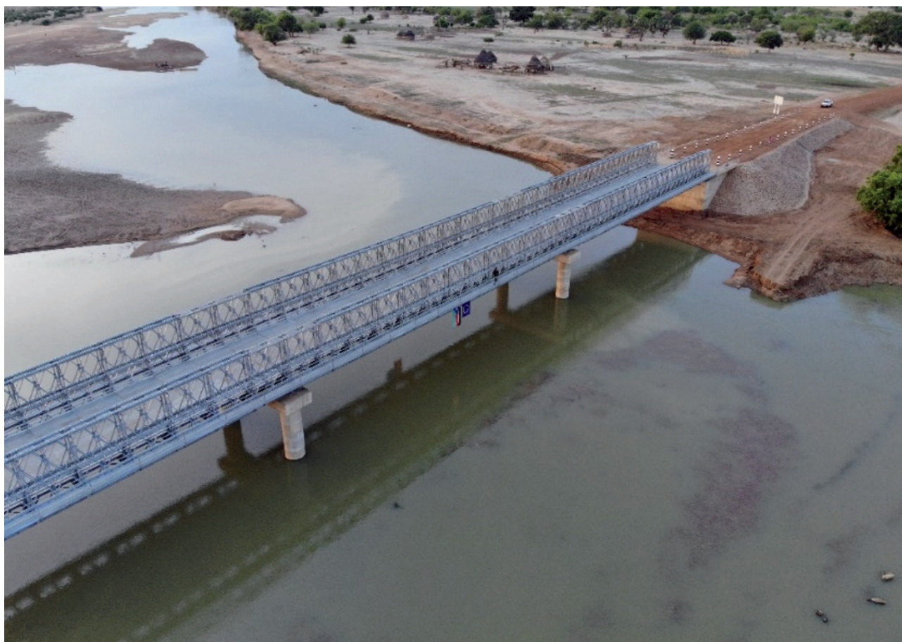
Figure 2: Kuajok Bridge in South Sudan built by WFP Engineering. This bridge proved essential in the transport and delivery of humanitarian assistance during the multi-year flooding event affecting the country. Photo: WFP/Country Office Engineering team
