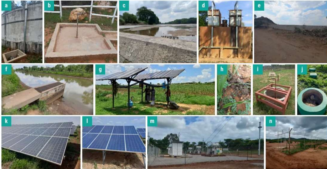
Figure 8: (a) Ongoing expansion of Esigodhini water treatment and supply system; (b) a private sector-funded community water supply scheme; (c) a sand dam at Tuli; (d) a sand dam water treatment and supply system at Ntepe; (e) ongoing construction of the Tuli-Moswa Manyange multi-purpose dam; (f) a dam supplying water at Mzinyathini irrigation scheme; (g, h) a solar-powered, drip-irrigated and organic manure fertilized community food and nutrition garden at Esibomvu; biogas digesters (i) supplying fuel for cooking and treated manure at a livestock farm and (j) energizing at Gwanda Agricultural Show; and solar power farms (k) in construction at Richaw site in Gwanda, (l) energising Mashaba community, (m) energising Blanket (Caledonia) Mine, (n) and in construction at Intratek site in Gwanda.
