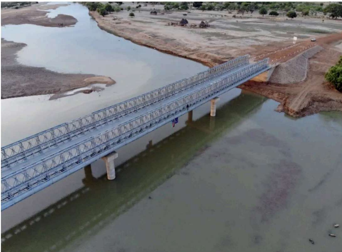
Figure 2: Kuajok Bridge in South Sudan built by WFP Engineering. This bridge proved essential in the transport and delivery of humanitarian assistance during the multi-year flooding event affecting the country. Photo: WFP/Country Office Engineering team
